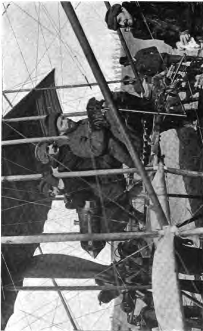
HENRI FARMAN WITH 2 PASSENGERS Note the control levers and wires leading to the rudders and ailerons.
